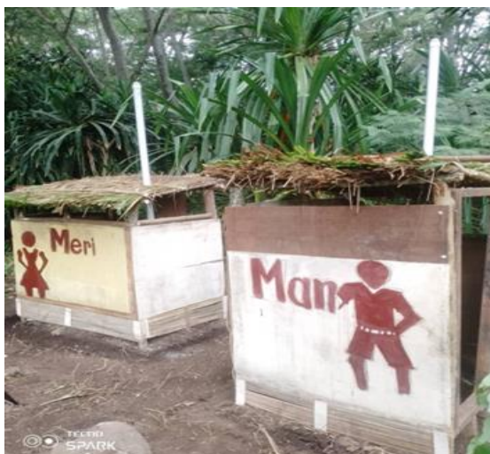
Figure 6: Construction of latrines at the Evacuation Centre
