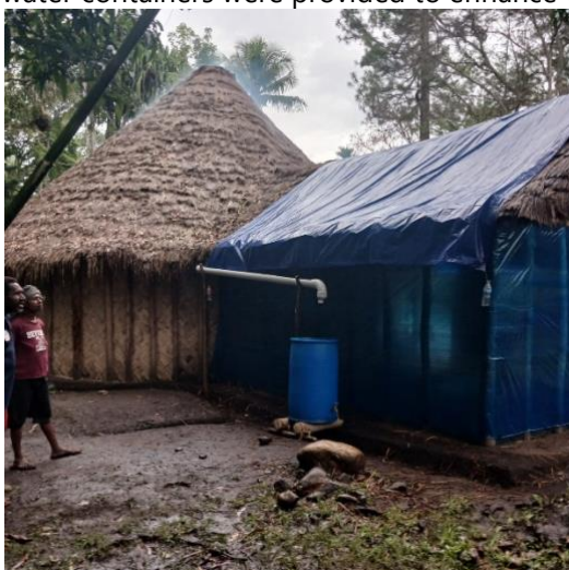
Figure 4: Temporary water harvest system #1
