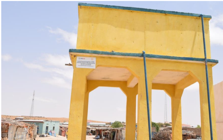
Photo 2. Water Tank Constructed by STORRE in Carmale Village
