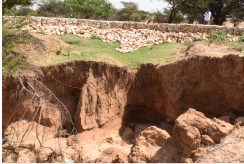
Photo 3. Gabion built to control Gully Erosion in Jiidali Village
