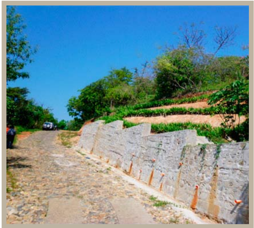
Slope stabilisation demonstration project using vegetated terraces
