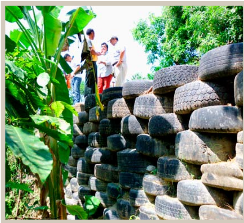
Contention wall demonstration project, built according to the community's own initiative using recycled tyres to stabilise the slope in San Bernardo Guatemala
